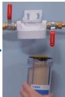
► Remove the used cartridge from the bowl and position the new cartridge without worrying about the direction of orientation. Pay attention to the correct positioning of the black seal which must not be pinched.
